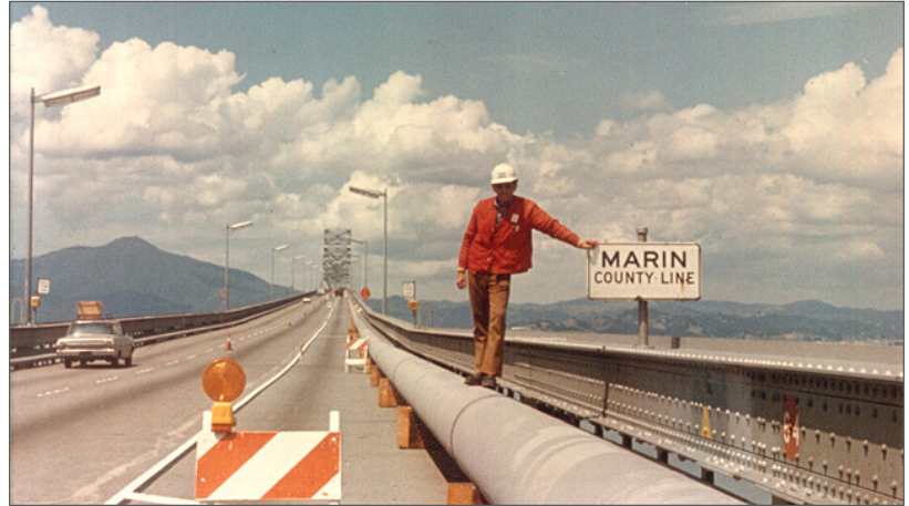
Emergency pipeline, San Rafael Bridge (1977 drought)
